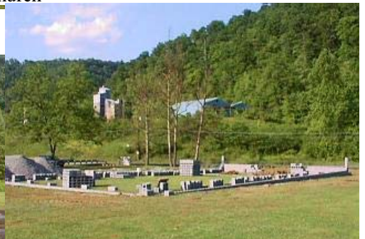
First Blocks Laid For Foundation.
