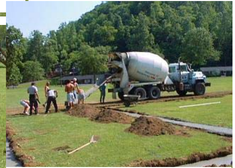
First Cement Poured For Footers
